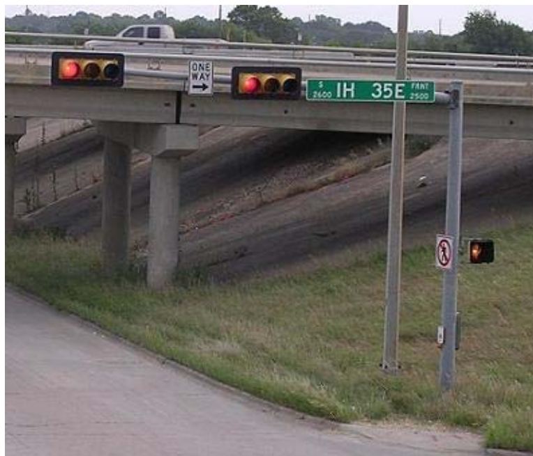
Figure 1.1.1 Typical Cantilever Traffic Signal Structure
