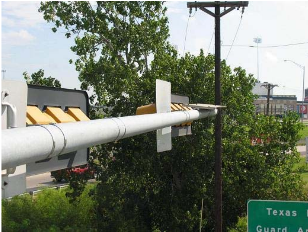
Figure 6.2.4 Horizontal Damping Plate on Mast Arm 2
