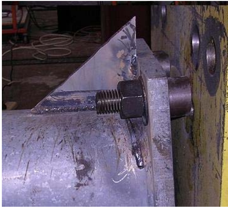
Figure 8.3.4 Stiffener Added to Mast Arm DU After 116,876 Cycles
