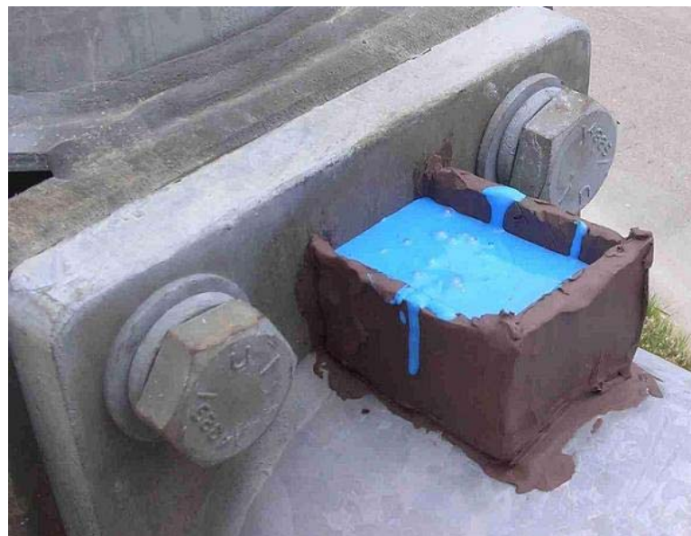
Figure 2.3.2.1 Clay Dam Filled with Molding Material
