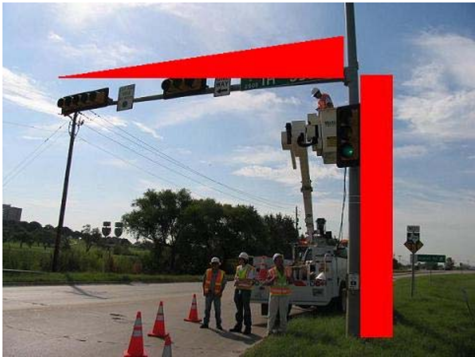
Figure 2.1.1 Moment Diagram Superimposed on Cantilever Mast Arm
