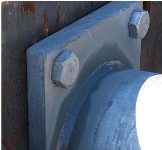
Figure 5.3.4.2 Drying Zinc-Rich Paint
