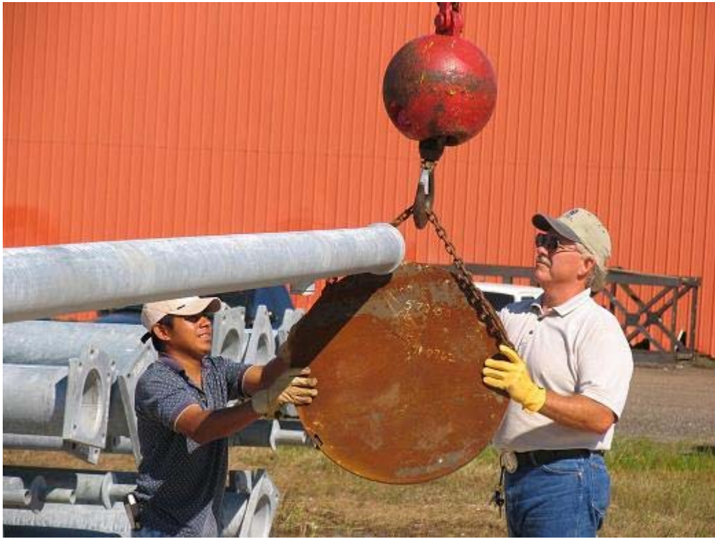
Figure 5.3.1.4 Placing the 500-Pound Circular Weight on the End of the Mast Arm
