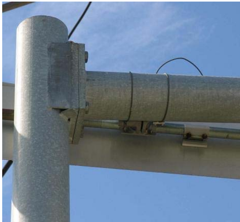
Figure 1.1.2 Mast Arm Base Plate-to-Built-up Box Bolted Connection
