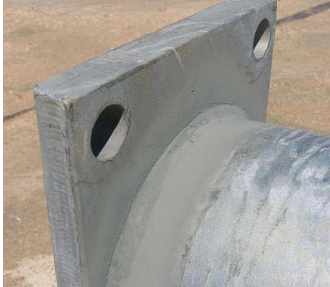
Figure 5.3.4.3 Mast Arm Weld After Completion
