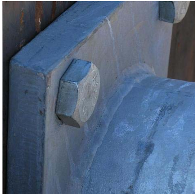
Figure 5.3.2.4 Mast Arm-Baseplate Weld Connection Before UIT Application
