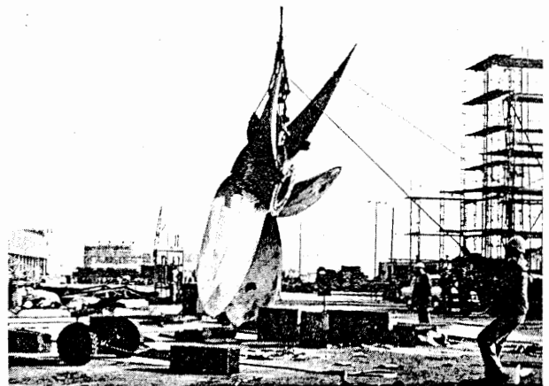
Fig. 4—Propeller being lifted into position
