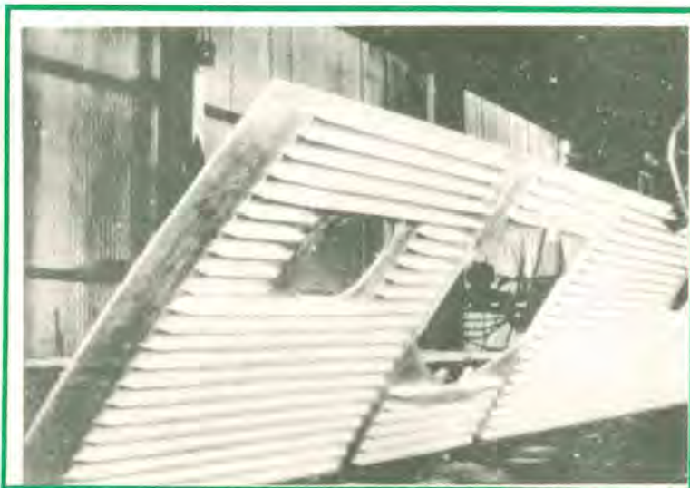
First peen formed integrally stiffened wing skins, for Lockheed Super-Constellation.
