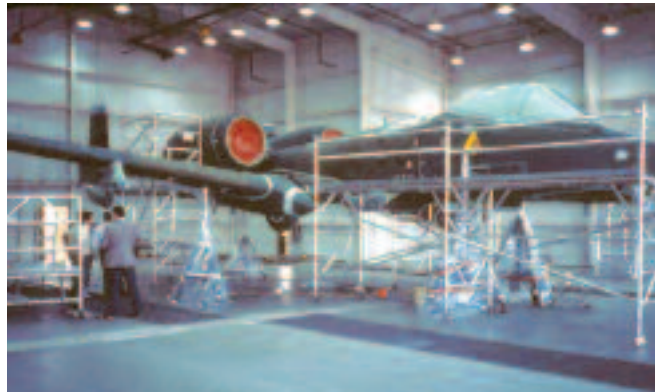
Aerolyte dry stripping facility for depainting A-10 aircraft at Hill Air Force Base, Utah.
