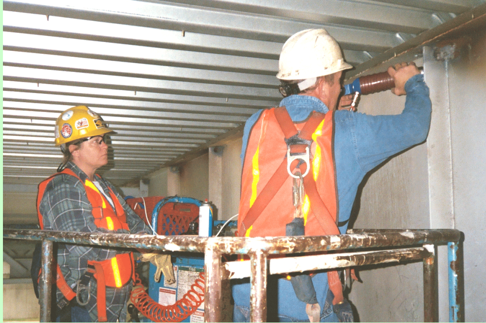
Ultrasonic Peening of welded elements of a highway bridge
