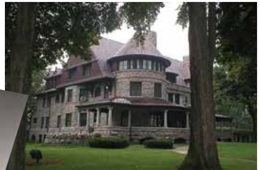
Copshaholm, built in 1895 and now a museum, was originally the home of J.D. Oliver, president of the Oliver Chilled Plow Works. The furnishings on all three floors are original, giving visitors a remarkable glimpse of how the Oliver family lived during their 72 years in the home. Copshaholm is within walking distance of the Marriott and the Century Center.
